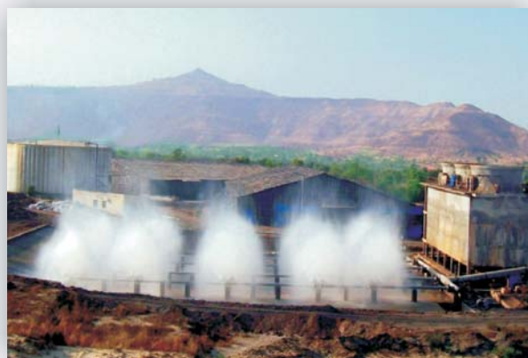
MCS replacing Cooling Tower
